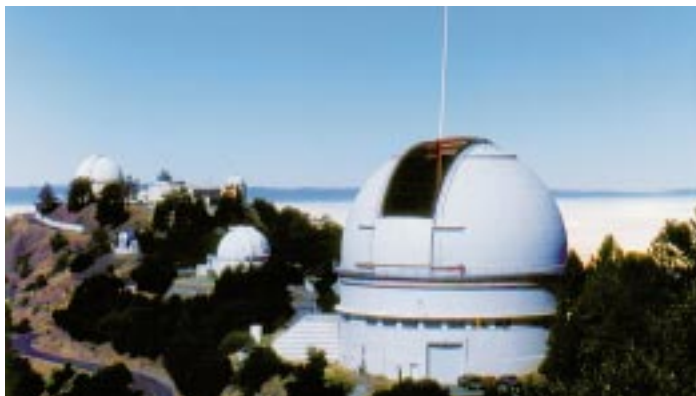
The adaptive optics system at UC's Lick Observatory uses a laser beam (captured in this time-exposure photo) to measure turbulence in the atmosphere.
